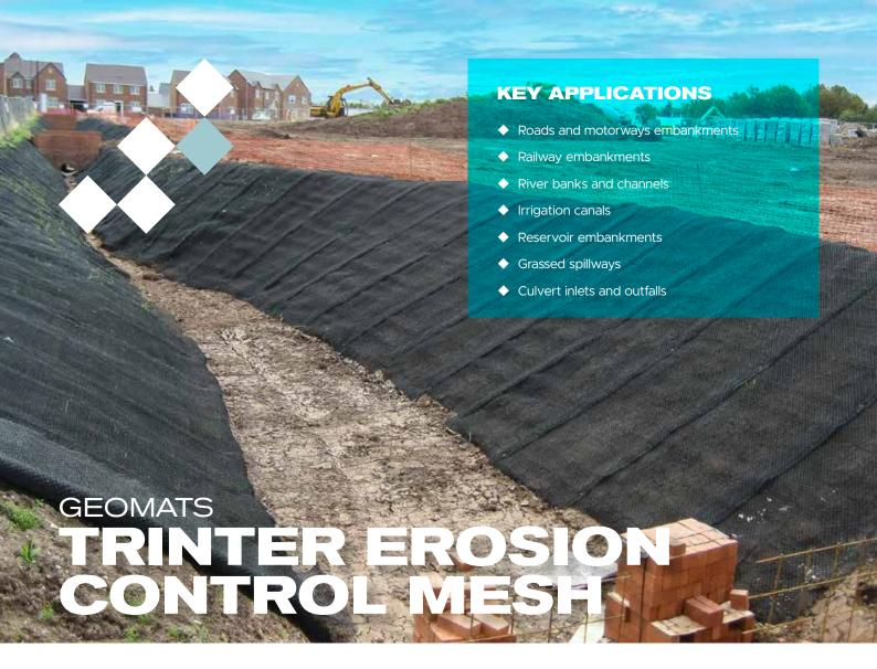
Erosion control on banks and slopes is a common problem faced by many contractors and engineers. Erosion control matting is used as a lightweight solution to help establish healthy vegetation for permanent erosion protection on banks and slopes.
