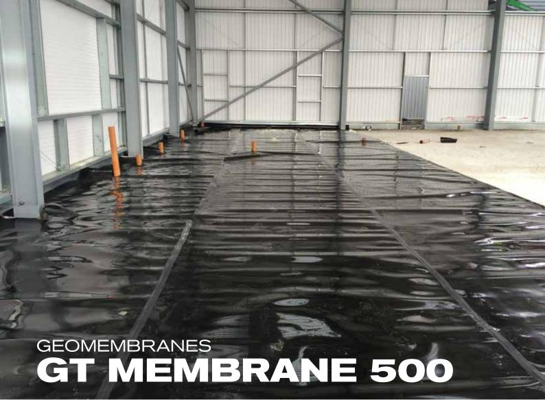
Our standard impermeable geomembranes are a popular choice for creating a watertight barrier to prevent storm water from filtering out and saturating the surrounding ground.
