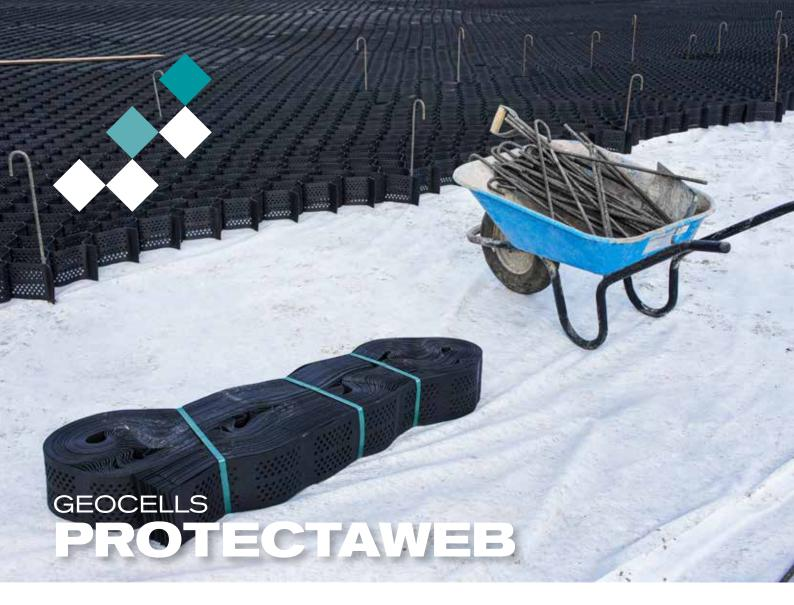
Our ProtectaWeb is an established and proven method of constructing access tracks or parking areas close to tree roots without causing them undue stress and possible damage.
